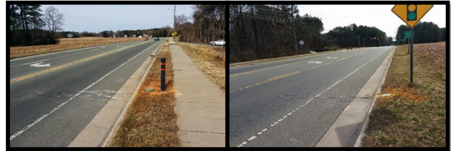
Figure 1. Continuous Count Station Installation East (Left) and West (Right)
