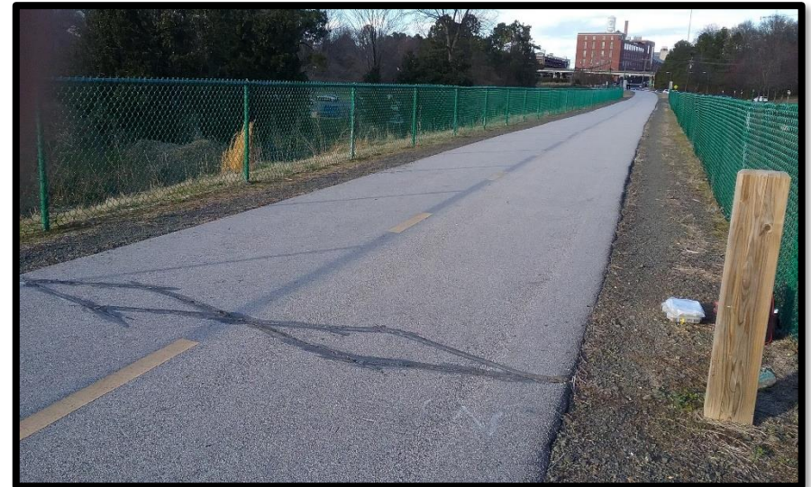
Figure 1. Continuous Count Station Installation West (Left) and East (Right)
