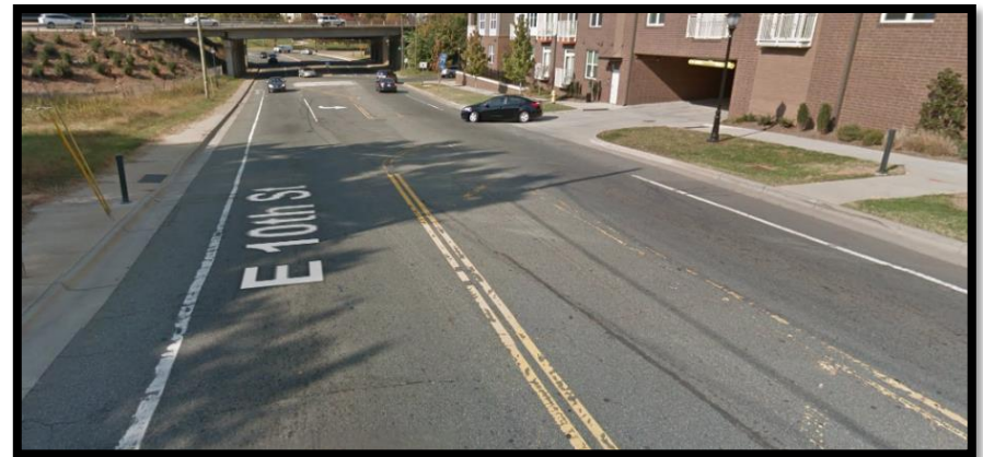
Figure 1. Continuous Count Station Installation
