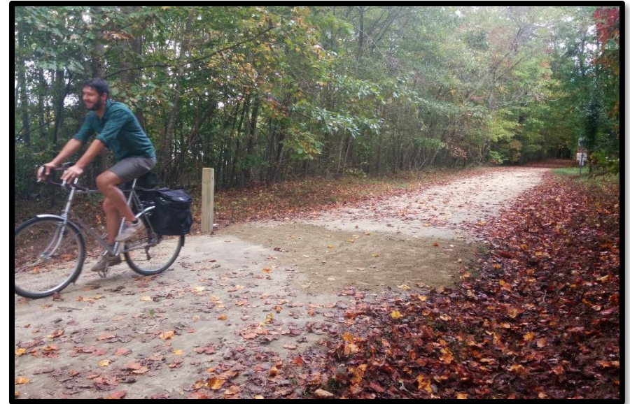
Figure 1. Continuous count Station Installation
