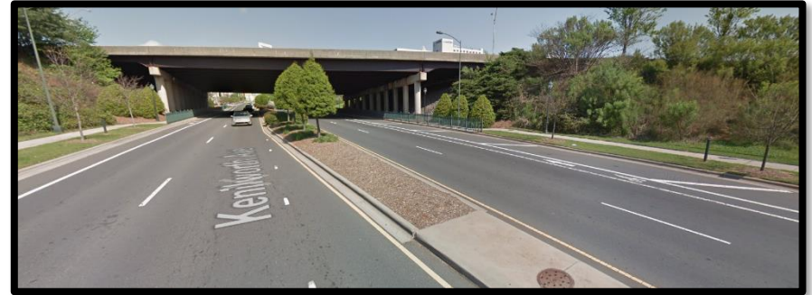
Figure 1. Continuous Count Station Installation
