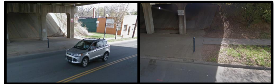
Figure 1. Continuous Count Station Installation North (Left) and South (Right)
